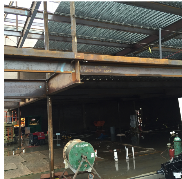
Metal Decking in Area C South Classrooms
