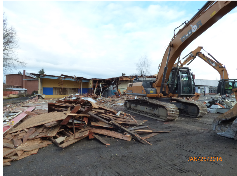
Faubion School Demolition
