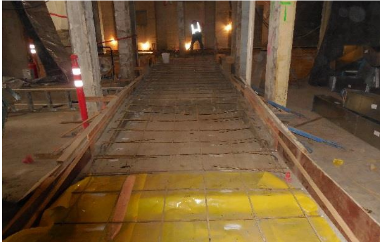
Auditorium Lower Level Ramp Formwork
