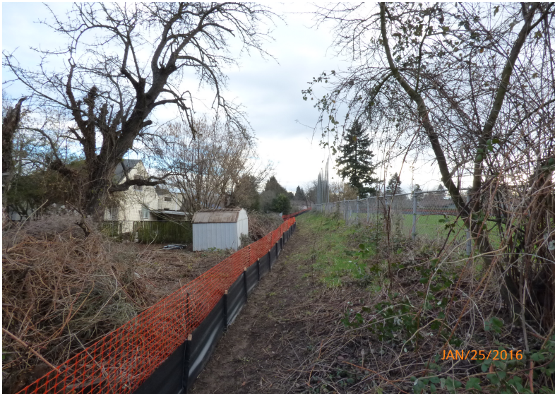
Silt Fence Installed on Perimeter
