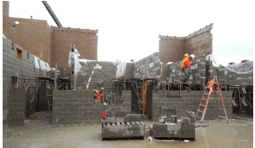
Locker Room CMU Wall Construction
