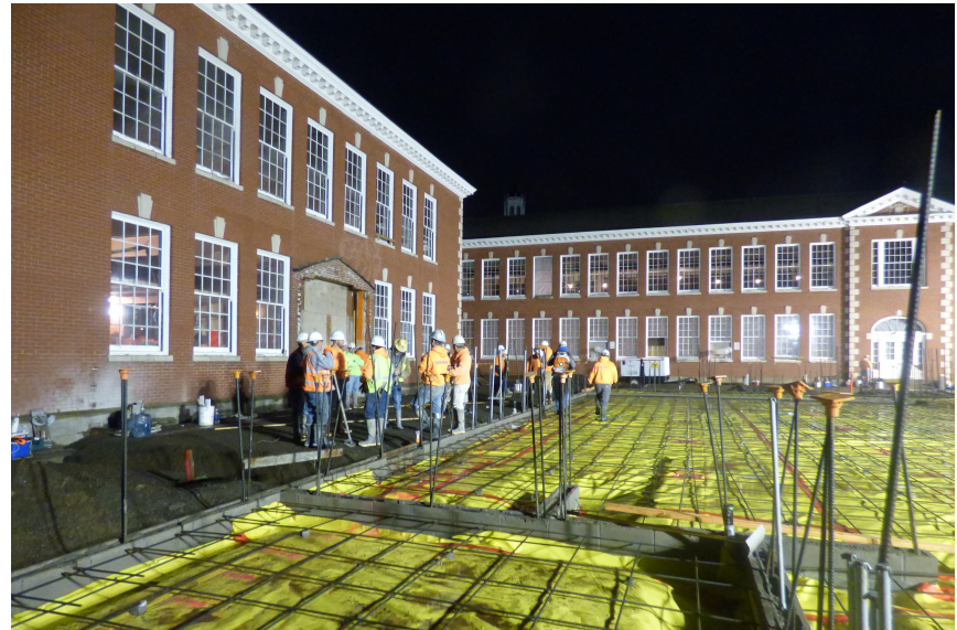
07:00 AM Concrete Placement Prep
