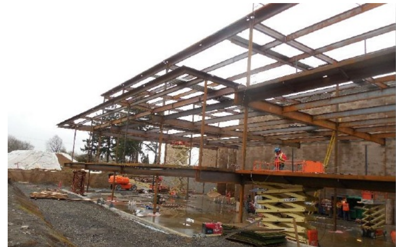
Area C Structural Steel
