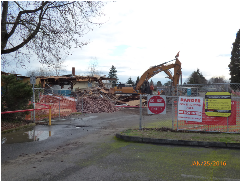
Active Demolition Site
