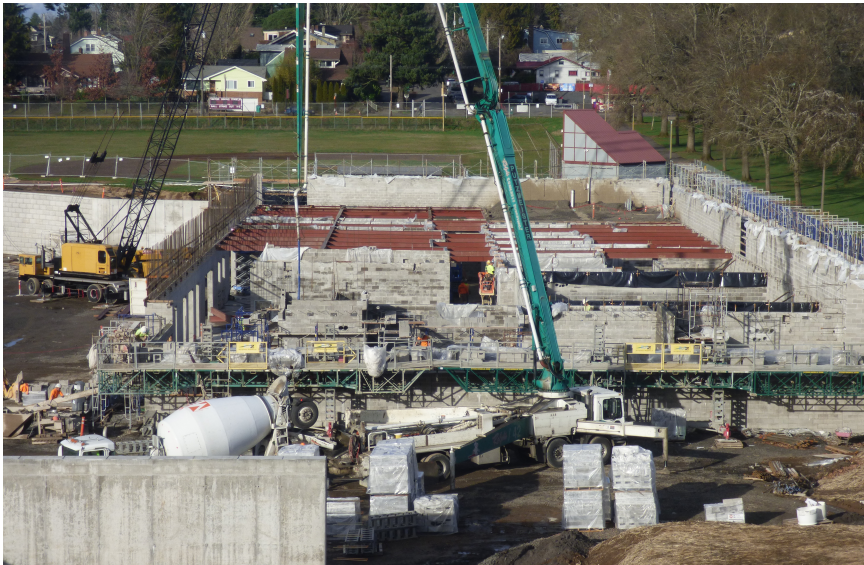
Progress on New Gymnasium
